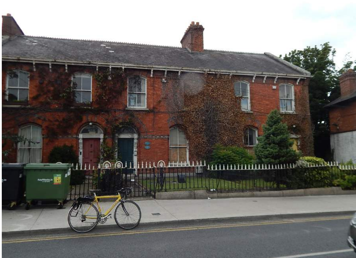
Photograph: Glenville Terrace, 2017
