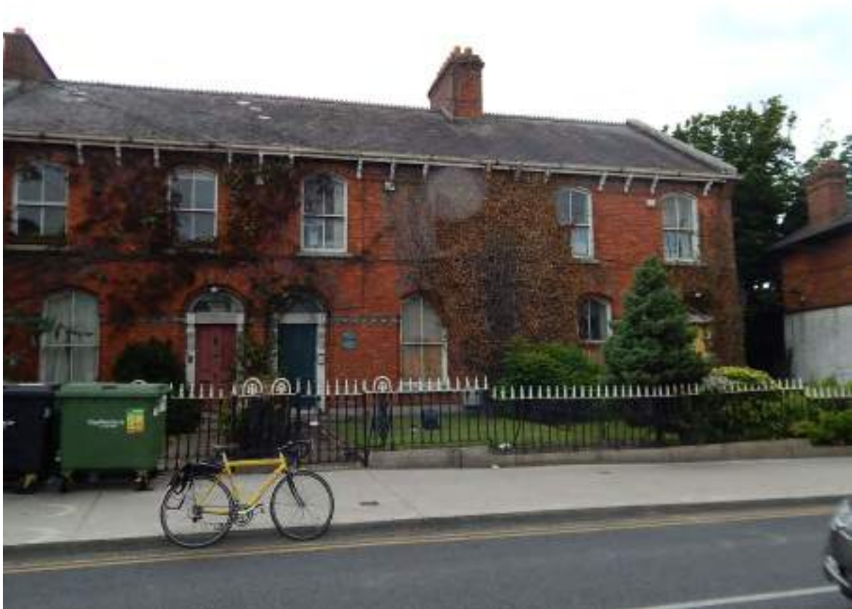
Photograph Glenville Terrace
